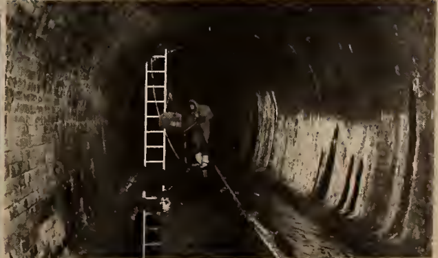
Studying the Stoney Brook Culvert.*
